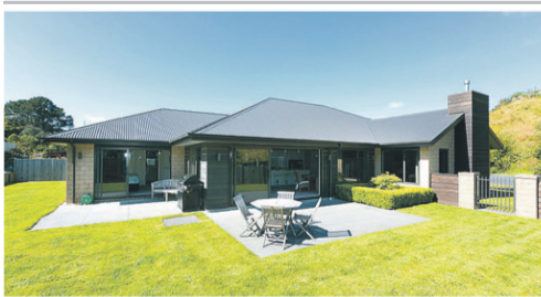
Hurworth 11 Fernbrook Drive
